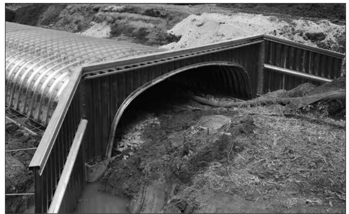
ALBC with headwall and wingwalls.
