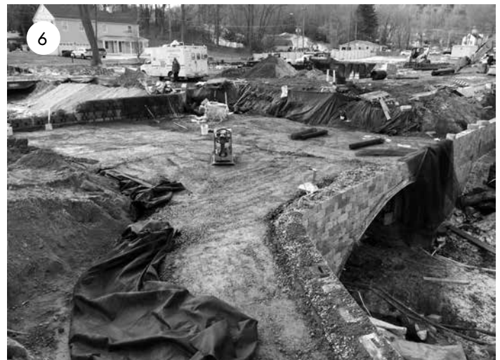
Compact material with a vibratory plate compactor.
