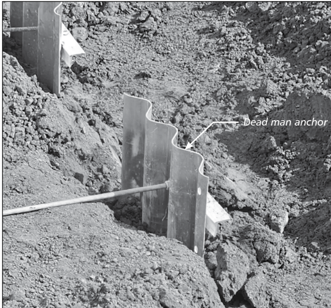
Attaching deadman anchor to 3/4" threaded tie rod.
