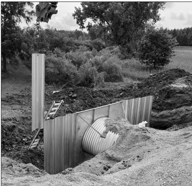
Sliding 7-gage hot-dip galvanized sheeting into place.
