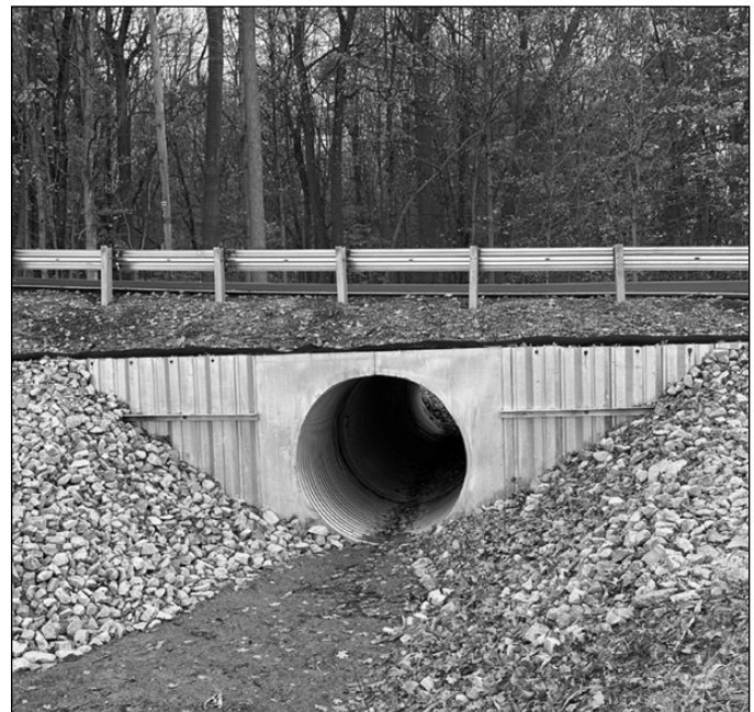
Completed headwall with wingwalls.
