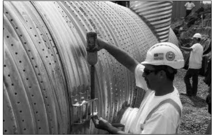
Tightening bolts on a corrugated band.
