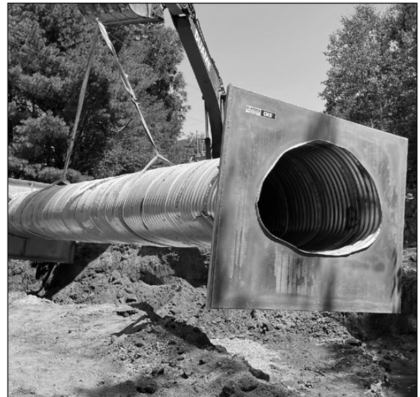
Lifting single piece with two nylon straps.
