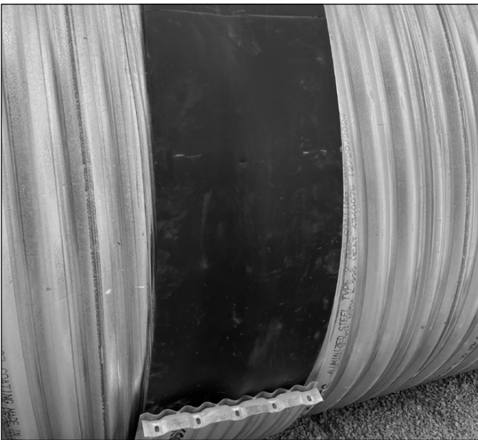
24 inch wide flat neoprene gasket placed before band
