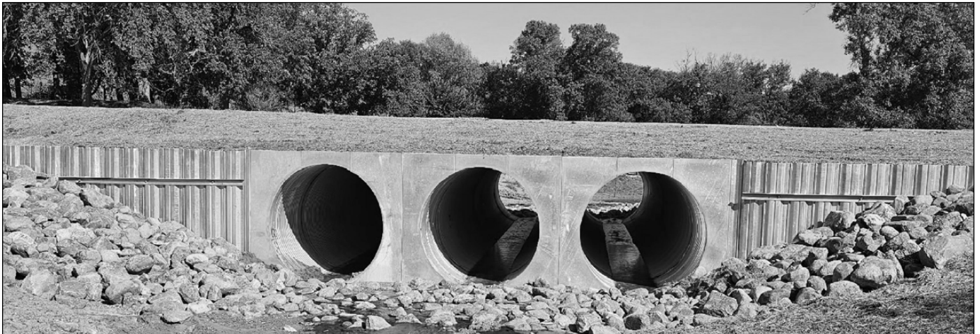
Completed CHS project.
