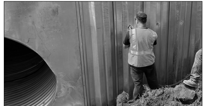
Blowing one inch holes in sheeting to place anchor rods.
