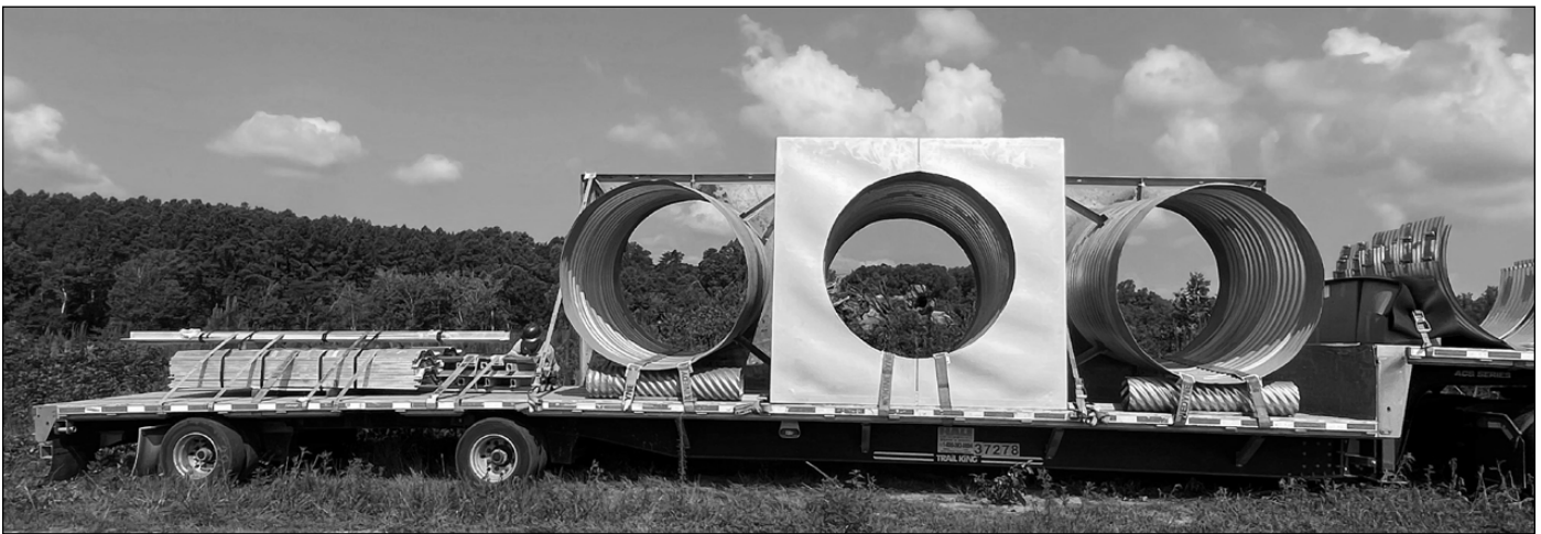
Large diameter CHS arriving to project site on flatbed trailer.
