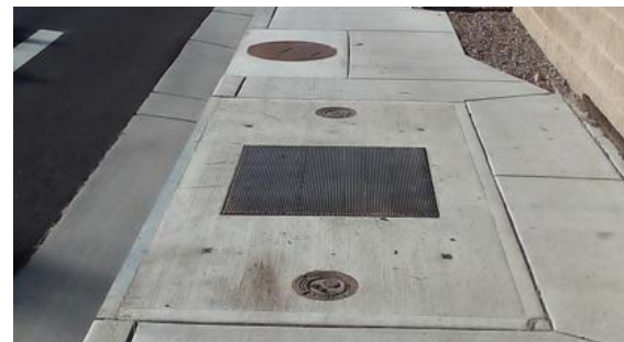
Figure 2b. Filterra with Full Grate Photo
