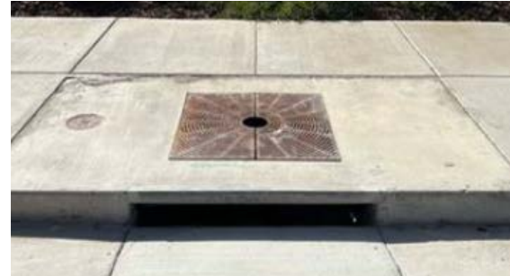
Figure 1b. Filterra with Tree Grate Photo (not yet planted)
