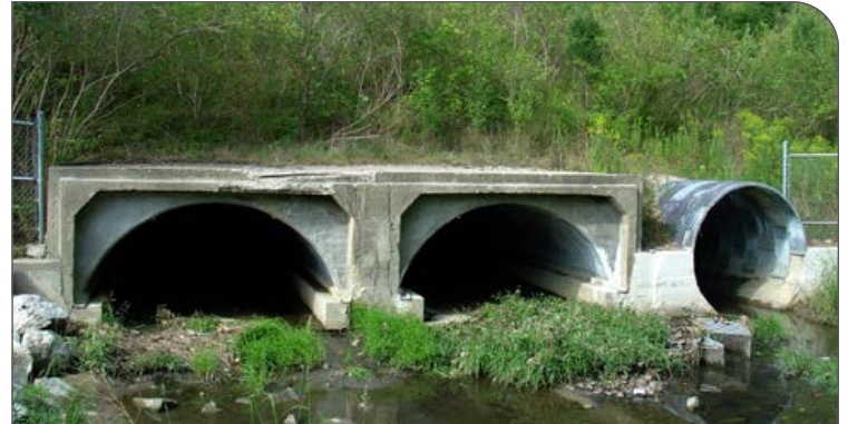
I-675 Culvert Reline, OH – provide optimum shaft stability and protection relining structures under roads (Tunnel Liner Plate)
