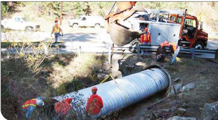
Brook Forest Road Cross Culvert, CO – reline aging culverts to provide exceptional flow and structural integrity (ULTRA FLO®)
