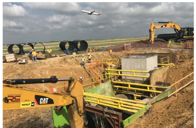
DuroMaxx® SRPE is an extremely efficient solution for glycol storage able to handle the heavy live-loading of an Airbus A380.
