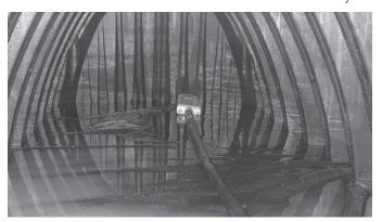
The tool will backflush the Containment Row forcing debris into the diversion manhole sump. Use the stringer vacuum hose to remove the sediments and debris from the sump of the diversion manhole. Multiple passes may be required to fully cleanout the Containment Row. Vacuum out the diversion manhole and remove all debris. See Figure 1.
