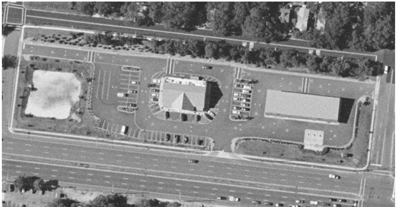
Figure 2 Aerial view of WAWA Market Route 37 study site
