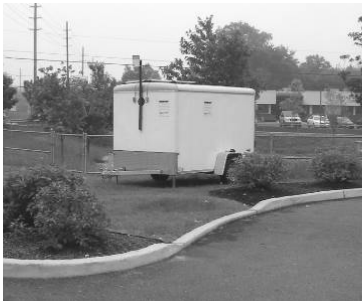
Figure 5 View of the Mobile Monitoring Unit (MMU) installed at the WAWA Market Route 37 study site
