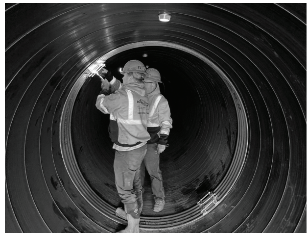
Above: Corrugated Steel Internal Band with Angles
