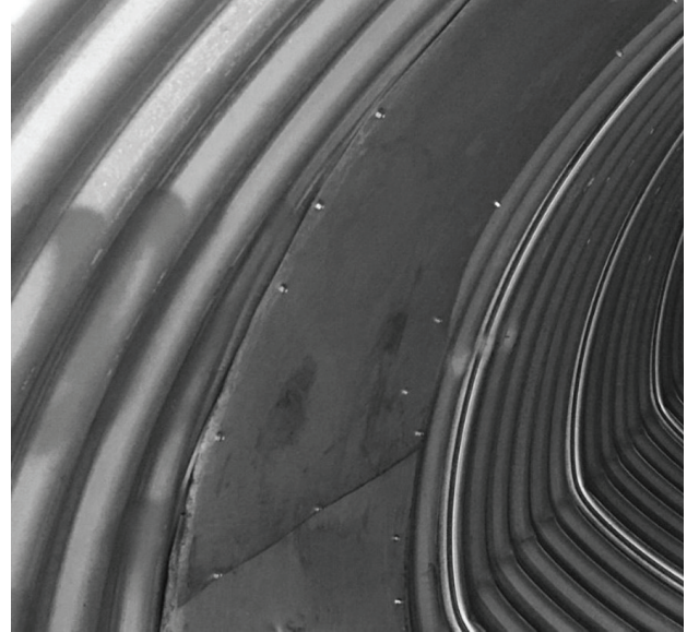
Above: Flat steel band with self-tapping screws
