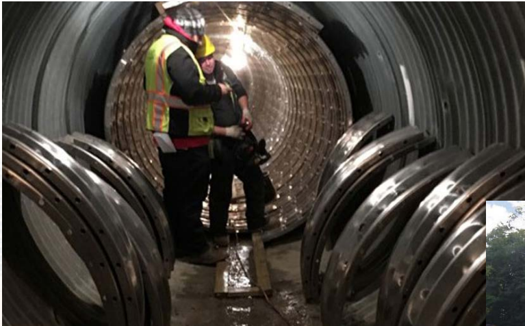
CONTECH® 2-FLANGE TUNNEL LINER PLATE
