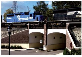
Railroad Overpass — Precast arch units support railroad loading over a roadway underpass.
