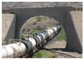
BridgeCor® structural plates unique corrugation allows for spans of up to 60 feet – ideal for railroad underpasses or large clearance areas.
