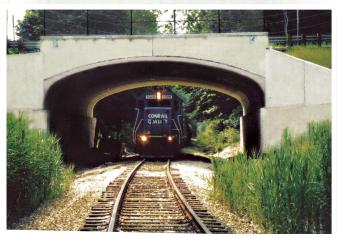
Railroad Underpass — Precast arch units provide a perfect solution to vehicular/pedestrian access roads over railways.
