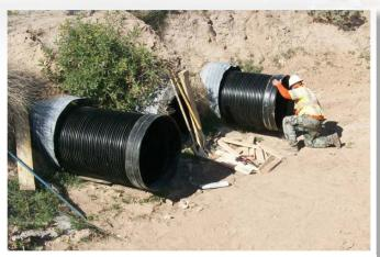
$\label{lem:condition} Duro Maxx\ Steel\ Reinforced\ Polyethylene\ (SRPE)\ pipe\ is\ slip\ lined\ to\ provide\ a\ structural\ lining.$
