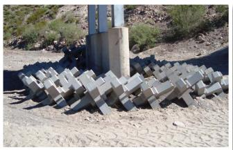
A-Jacks articulating concrete blocks are an excellent solution for scour protection around piers and bridge structures.
