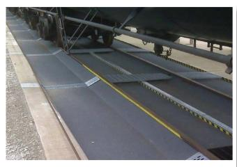
Collector Pans — Provide the ideal solution to control spills at fueling stations.
