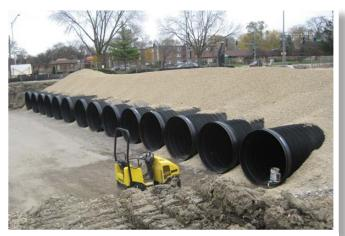
DuroMaxx Steel Reinforced Polyethylene (SRPE) pipe.
