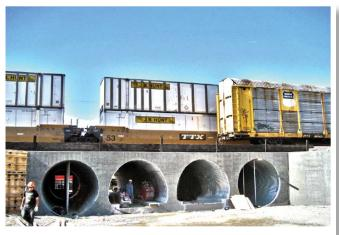
MULTI-PLATE® offers a wide range of shapes and sizes for specific site considerations – pipe arch with concrete paved inverts shown.
