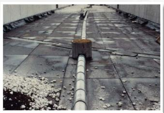
Use Contech Deck Drain to collect and transport water from the surface of the rail road bridge.
