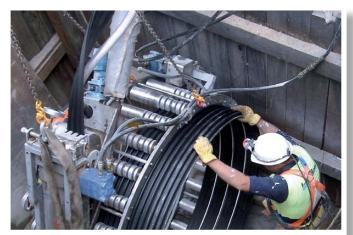
$SPR^{TM}$  PE is a spiral wound, steel reinforced HDPE that is heat-fused to form a structural pipeline rehabilitation product.
