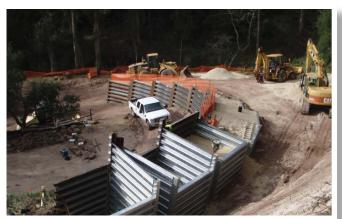
Retaining Walls — Bin-Wall is a lightweight steel that is easily assembled to fully enclose fill material for a solid wall solution.
