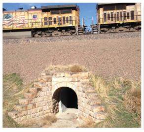
Contech Tunnel Liner Plate was used to fully restore this pedestrian underpass directly under a fully operational rail line.
