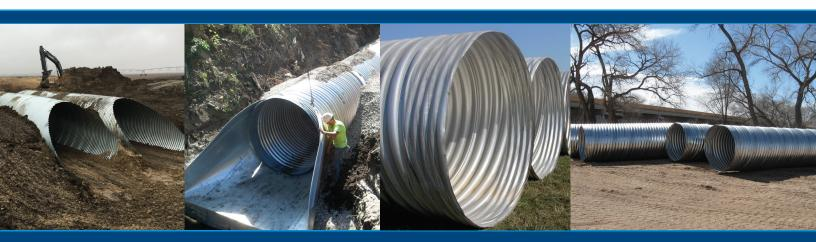
3x1 and 5x1 corrugations for manufacturing of Corrugated Steel Pipe are considered to have **equal "stiffness"** in the industry. 3x1 tooling was first developed and later 5x1 (metric dimensions) tooling was made available in the industry.
