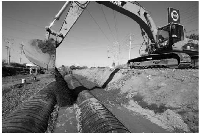
ULTRA FLO® can be manufactured from polymer coated steel for added durability.
