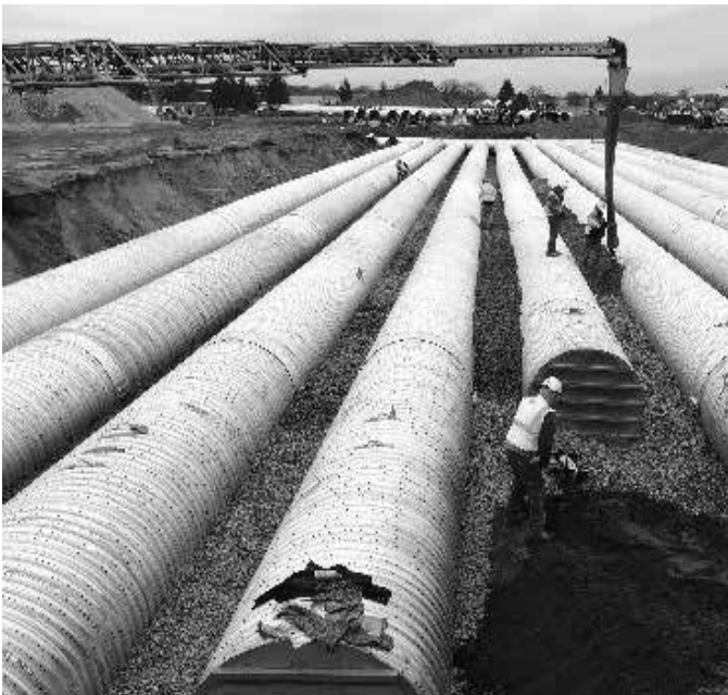
Placing backfill with a conveyor.
