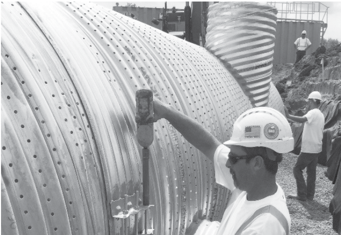
Tightening bolts on a corrugated band.
