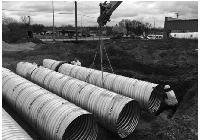
Lifting ALT2 CMP with nylon slings.
