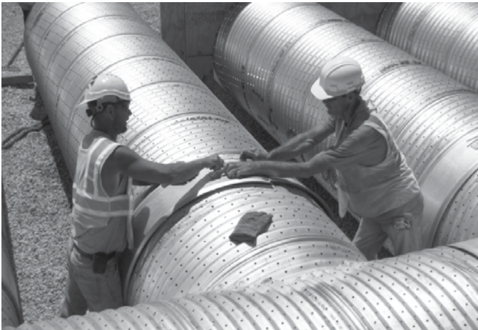
Installing a Hugger band on a perforated pipe.
