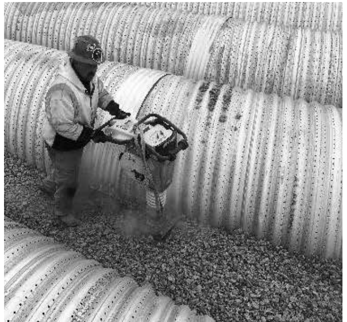
Compaction with vibratory equipment.
