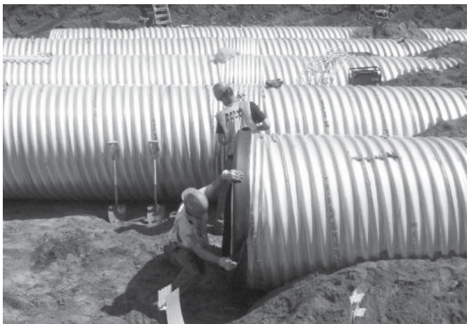
Installation of band with flat neoprene gasket.
