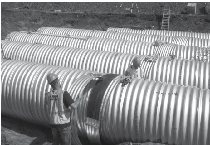
Tightening bolts on a corrugated band.
