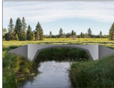
BURIED BRIDGE – Bottomless structure surrounded with soil.
