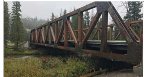
Steadfast Vehicular Truss with Big R Rolled Girder Approach Spans
