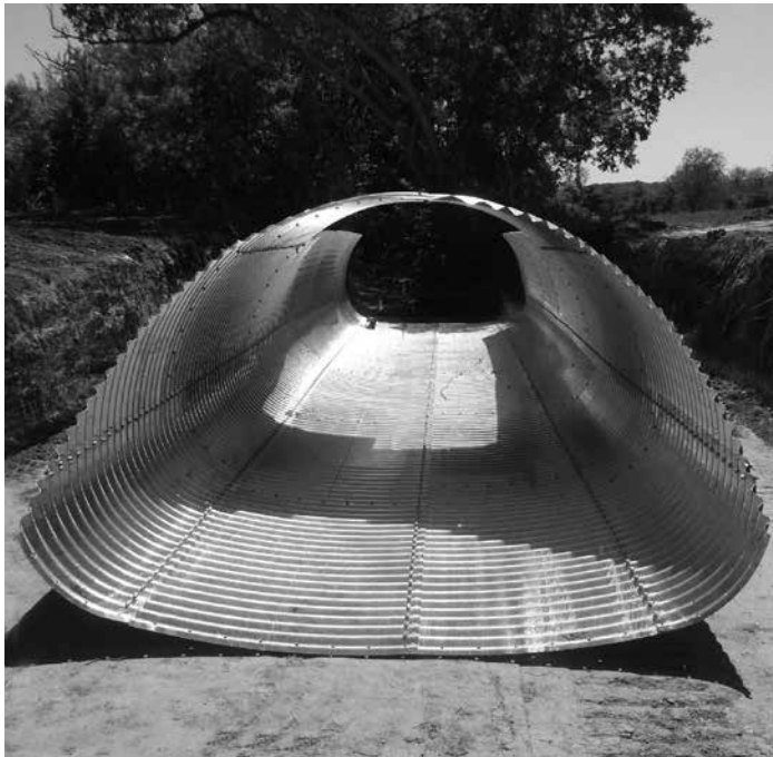
Typical End View of a Pipe-Arch with a Step-Beveled End
