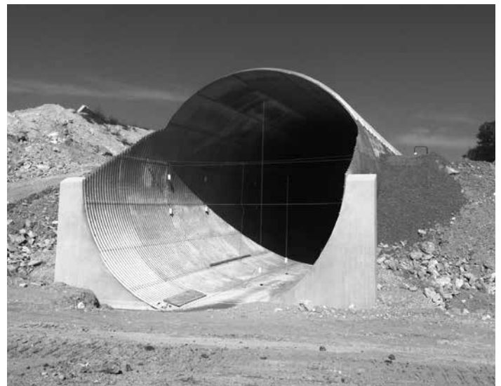
Cast-in-Place Toewall
