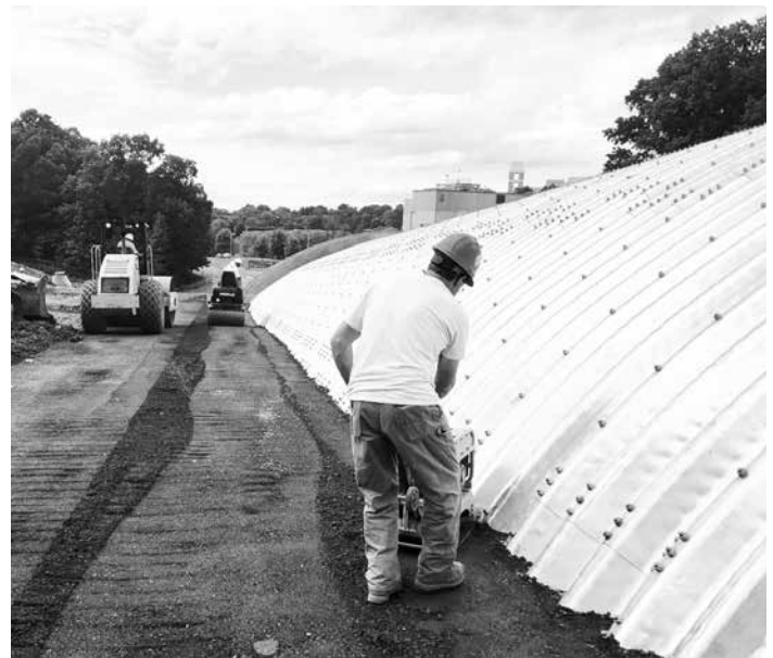
Figure 13. Adequate, uniform compaction is critical to building soil/steel structures.
