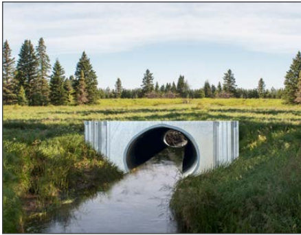
CULVERT – Structure with an invert encompassed with soil.
