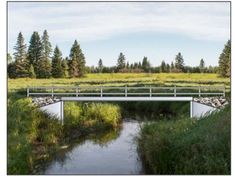
BRIDGE-AT-GRADE – Structure that clear spans from embankment to embankment.
