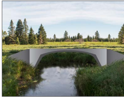
BURIED BRIDGE – Bottomless structure surrounded with soil.
