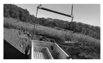
It is the contractor's responsibility to provide suitable lifting equipment to offload the Contech vault. Contech vaults are designed to be offloaded using the contractor's spreader bar.
