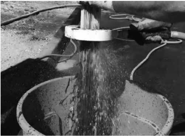
Rinsing Cartridge with Contech Rinse Tool
