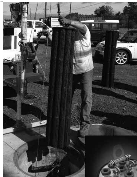
Cartridge Removal & Lifting Device
