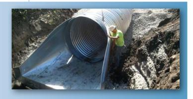
With over 100 years of proven performance, Contech corrugated metal pipe (CMP) solutions offer the best combination of pipe strength and economy for culverts and storm sewers. CMP is available in round and pipe-arch shapes up through 144" diameter and can be manufactured with helical, lock-seam construction or annular corrugations with riveted or spot welded seams. A variety of coupling systems are available to meet the project requirements.
