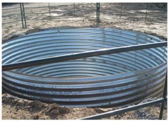
CMP is used as a deep foundation form at the base of the windmill
