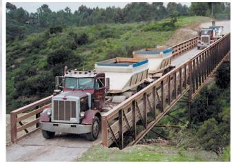
Steadfast® vehicular truss structures are an economical design solution because of the high strength-to-weight ratio of steel
