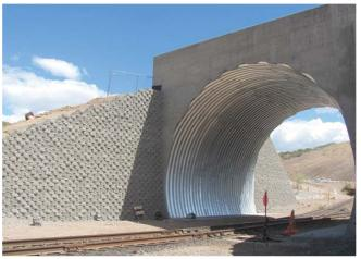
BridgeCor® structures enhance the established performance of  $6'' \times 2''$  MULTI-PLATE by offering 9 times the stiffness and 3 times the strength
