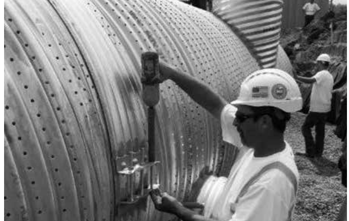
Tightening bolts on a corrugated band.
