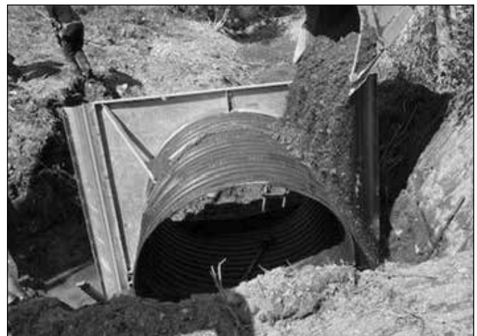
Placing a dense graded aggregate (DGA) behind the headwall.
