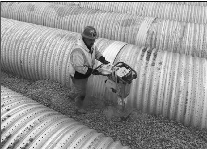
Examples of compaction with vibratory equipment around the culvert pipe.
