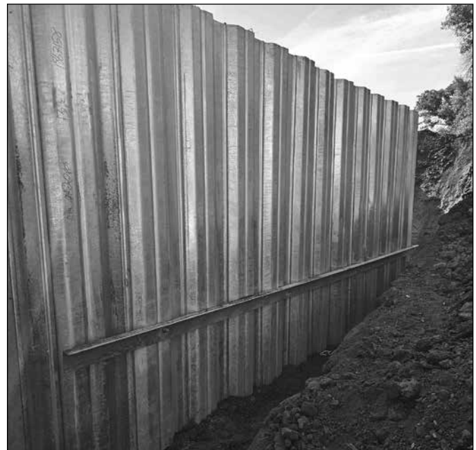
Close up of wale beam shown in front of the wall.
