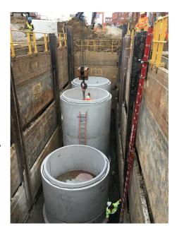
Installation occurred in two phases: the CDS manhole sections and the internals. First, the CDS manholes were installed; each consisted of a base slab, three barrel/riser sections, and a top slab. The fiberglass internals and screen were then installed by a Contech representative. Contech provided installation oversite and guidance to the contractor throughout the entire installation process of the CDS units.
