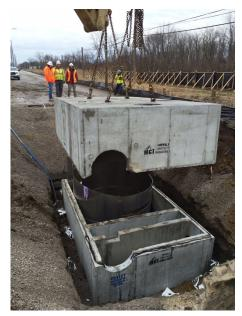
The Vortechs was chosen for this application because it can handle flows from a 100-year storm as well as act as an oil/grit separator for the access road, treating the water before it is eventually discharged into the Detroit River.
