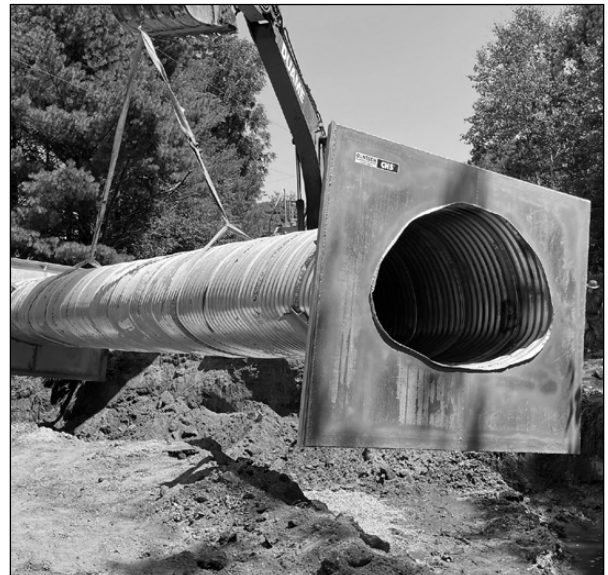
Lifting single piece with two nylon straps
