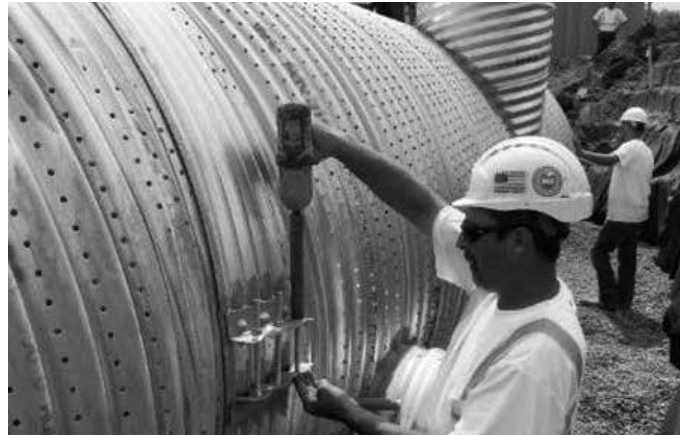
Tightening bolts on a corrugated band.
