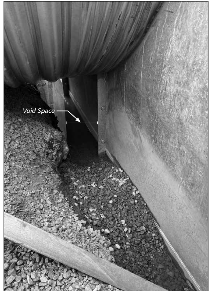
Void space under pipe needs to be filled with aggregate bedding material and compacted.
