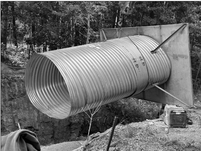
Lifting headwall with pipe stub with chains
