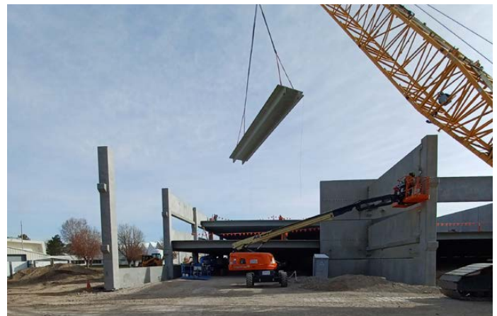
Erecting Precast Member
