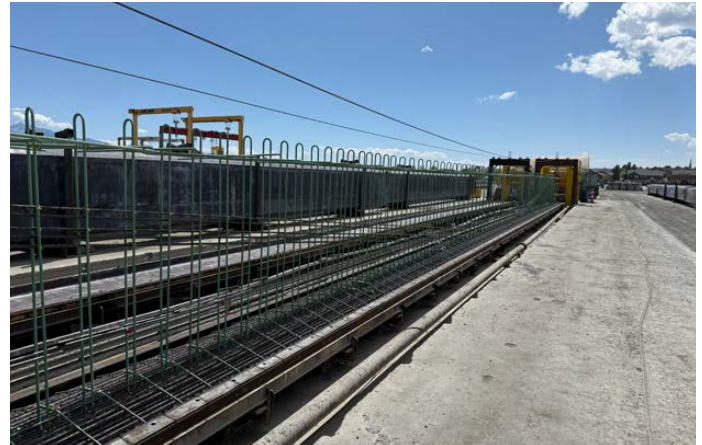
Placement of Reinforcing
