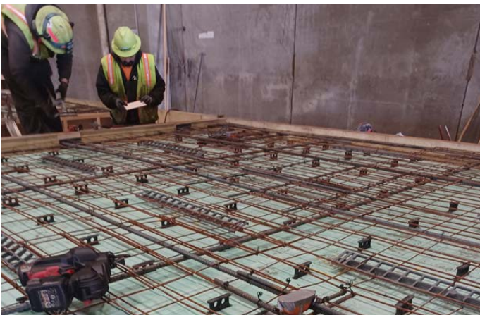
Embedded Items & Form Work
