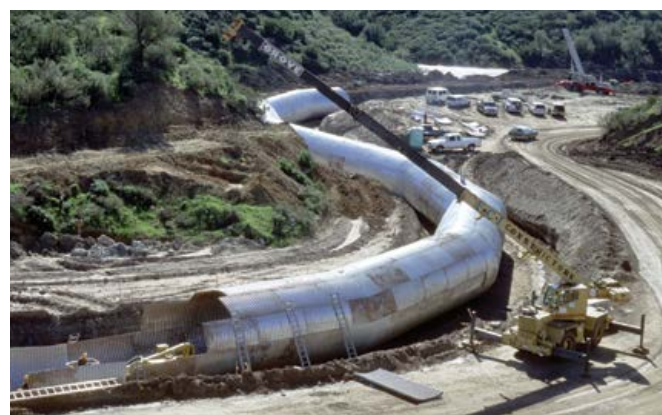
Structural Plate installed along curved alignment.
