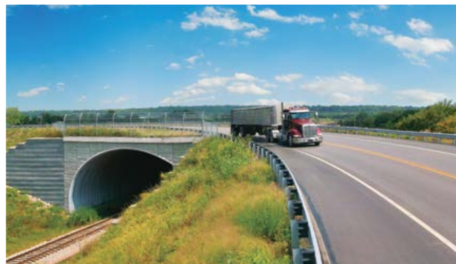
Contech's Structural Plate is ideal for grade separation and tunnels.
