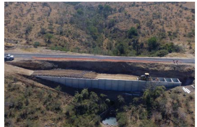
Bin-Wall provides an economical, gravity-type retaining wall solution.
