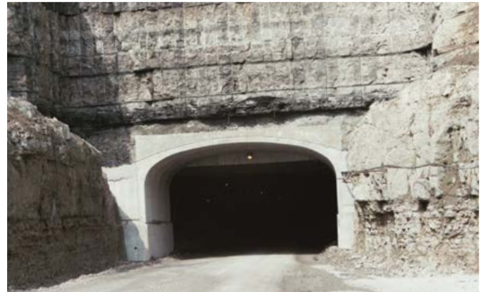
CON/SPAN precast arches can be utilized as portal protection.
