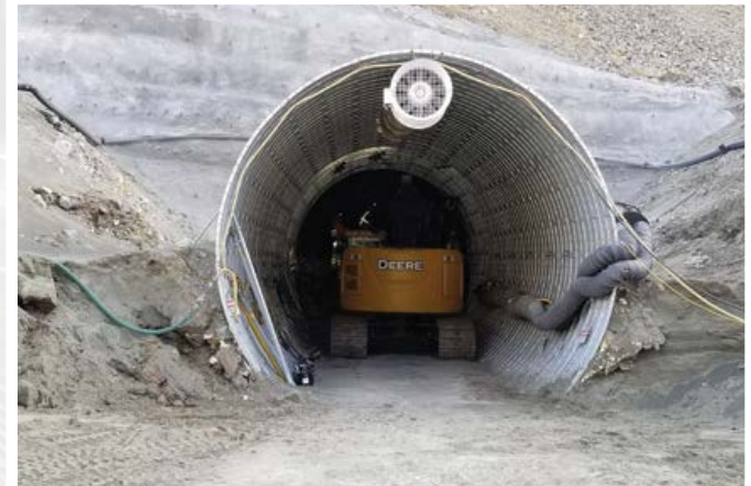
2-Flange Liner Plate offers superior plate stiffness and seam strength and the ability to construct from inside the structure.
