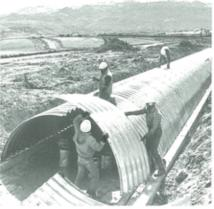
In-place structure assembly often negates the need for conventional lifting equipment.
