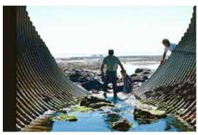
This aluminum structural plate pipe has handled tidal ocean waters under U.S. Highway 1 at the Bay of Fundy in Maine since 1966.
