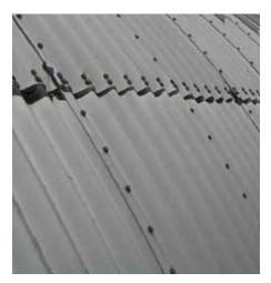
Plates are positioned by hand are ready for assembly.
