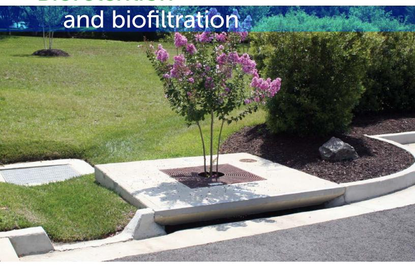
Bioretention and biofiltration use the physical, chemical and biological mechanisms found in nature to capture and filter stormwater. Providing both water quantity and quality benefits, biofiltration is ideal for Low Impact Development (LID), Green Infrastructure, and Environmental Site Design projects. Plus, the presence of plants increases biological activity and enhances the appearance of your site.
