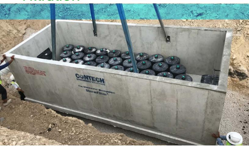
Stormwater filtration systems use media or membranes to remove total suspended solids (TSS), hydrocarbons, nutrients, metals, and other common pollutants from stormwater runoff. They can be housed in a vault, manhole, or catch basin and are used for both commercial and residential development, redevelopment, and stormwater quality retrofit applications. They can also provide pretreatment for Low Impact Development, infiltration, and rainwater harvesting systems.
