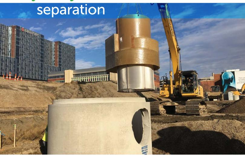
Hydrodynamic separators effectively remove sediment, hydrocarbons, trash and debris from stormwater runoff. These systems are often used as standalone and end-of-pipe treatment in both new and retrofit applications. They are also used as pretreatment to detention, infiltration, reuse and biofiltration to increase the service life of these systems by removing pollutants upstream.
