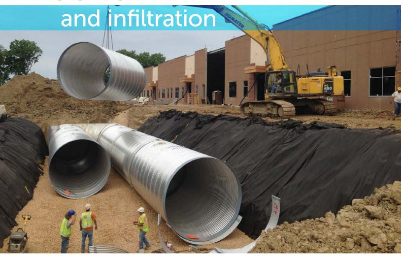
Detention and infiltration involves the use of vaults, chambers and pipes to temporarily store runoff. These structures often have open bottoms or perforations, allowing the excess water to be released slowly over time. In urban environments where there are competing demands for land, underground storage can provide many of the benefits of landscape-based systems but without requiring dedicated land area, thus maximizing the land value for the owner.
