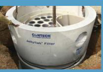
**SR-28 Improvements, Incline Village, NV:** A Jellyfish® Filter was installed to remove nutrients and fine sediment particles less than 16 microns to help improve the water quality of runoff entering Lake Tahoe.
