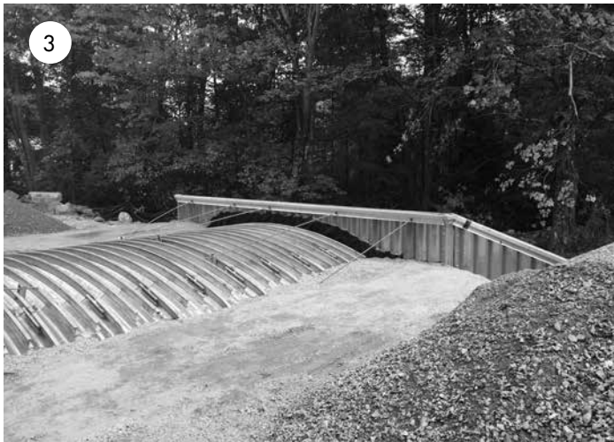
Granular material placed in balanced manner.
