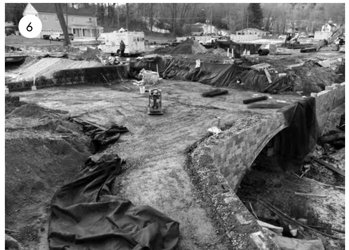
Compact material with a vibratory plate compactor.
