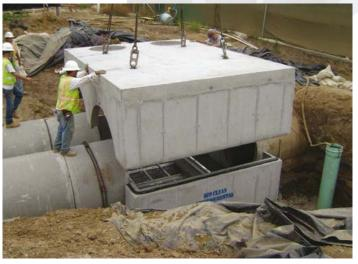
Units are frequently installed within a one-hour set time.
