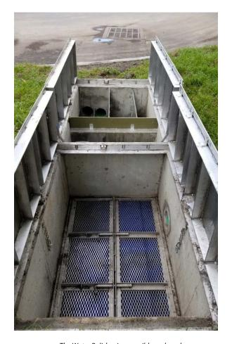
The Water Polisher is accessible and can be maintained from the finish surface.
