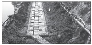
Float off concrete level with the top of foundation maintaining a level keyway. If applicable pour wingwall closure joints.
