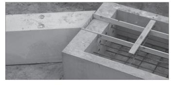
1. Set wingwall foundation flush with unit foundation using lifting points. Be sure to align threaded holes in the wingwall foundation segment with the openings in the end of the precast foundation segment.
