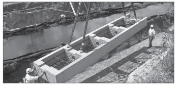
Attach foundation segment to the crane using preset lifting inserts in the precast foundation at all four locations. Slowly lower in to place taking care to line up correctly with the layout in Step I.
