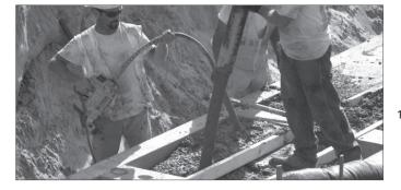
Block out vertical side of keyway using the proper size lumber to retain concrete infill and maintain the dimension of the keyway throughout the length of the foundation.
