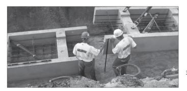
Match up connection at line and grade with the previous set segment making sure to leave 1/2" gap between segments per construction drawings.
