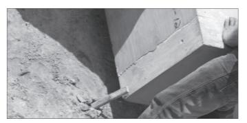
Stake the corners and use easily-visible string and marking paint to indicate the precise location to set the foundation according to construction drawings. Subgrade should be free of standing water.
