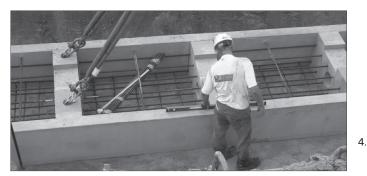
Verify each segment is set at proper elevation points prior to setting the next segment.
