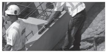
Check to make sure the segment is either level or sloped according to the elevation points in the construction drawings. Variations should not exceed 1/4" per ten feet. Place the subsequent adjoining foundation segments in the same fashion.
