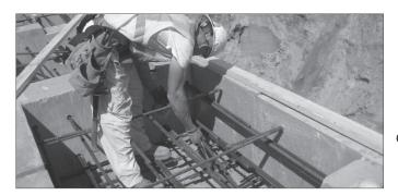
Prior to setting foundation segments for other side of bridge, verify span dimensions and elevations using laser measurements or other accurate method. Repeat as necessary with additional segments.
