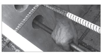
2. Use the supplied threaded dowels to connect the wingwall foundation to the unit foundation. Thread dowels into threaded receiver holes in wingwall foundation through open holes in the end of the unit foundation.
