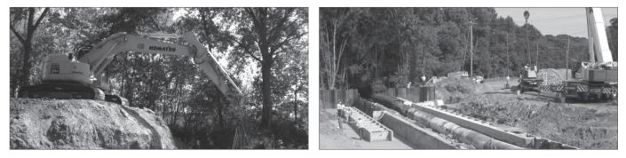
THE TIME OF THIS CONCRETE POUR WILL IMPACT WHETHER A GROUTING STEP IS NEEDED. THE CAST-IN-PLACE CONCRETE CAN BE POURED PRIOR TO SETTING THE STRUCTURE OR AFTER SETTING THE STRUCTURE.
