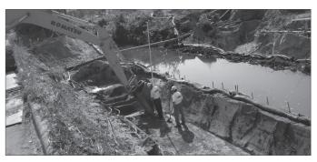
Excavate to the specifications in the construction documents. It is best to overexcavate the width a minimum 2' larger than the EXPRESS Foundation unit. In some cases a dense graded granular base material is specified as the leveling pad. Be sure to grade receiving pad +/- 1".
