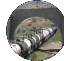
STRUCTURAL PLATE RAIL TUNNEL
