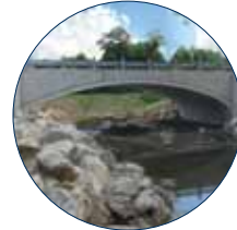
CON/SPAN PRECAST BRIDGE STREAM CROSSING
