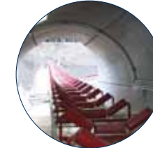
MULTI-PLATE RECLAIM TUNNEL
