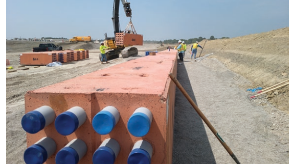
Patented shear key & joint system
