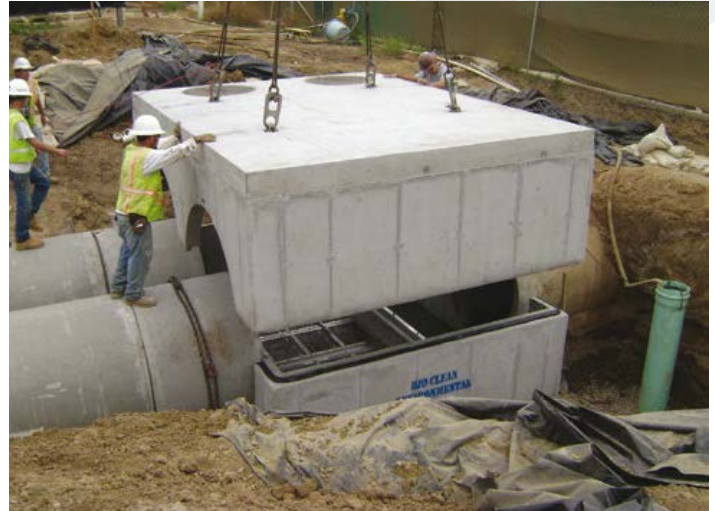
Units are frequently installed within a one-hour set time.
