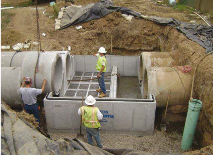
Shallow sump requires minimal excavation beneath the structure. Internal components are typically installed prior to delivery. Larger units may have internal components installed on site.
