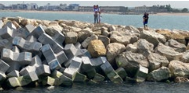
Figure 11-1: Transition between Xbloc and rock armour
