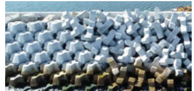
Figure 11-9: Transition between XblocPlus and Xbloc
