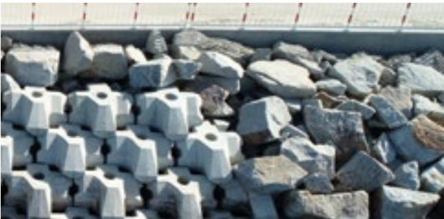
Figure 11-5: Transition between XblocPlus and rock armour
