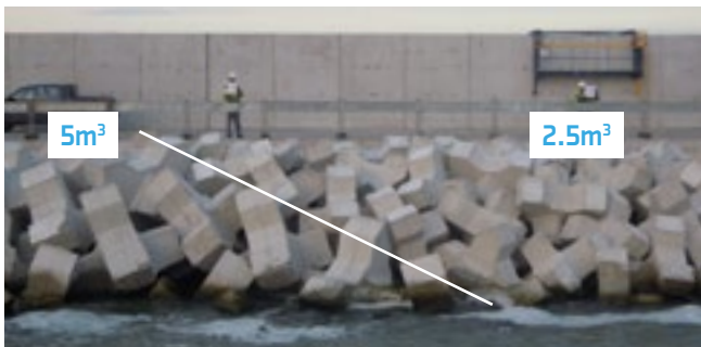
Figure 11-3: Transition between 2 sizes of Xbloc
