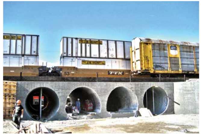
MULTI-PLATE® offers a wide range of shapes and sizes for specific site considerations – pipe arch with concrete paved inverts shown.
