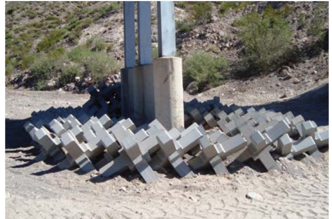
A-Jacks® articulating concrete blocks are an excellent solution for scour protection around piers and bridge structures.
