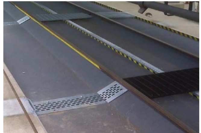
Collector Pans – Provide the ideal solution to control spills at fueling stations.
