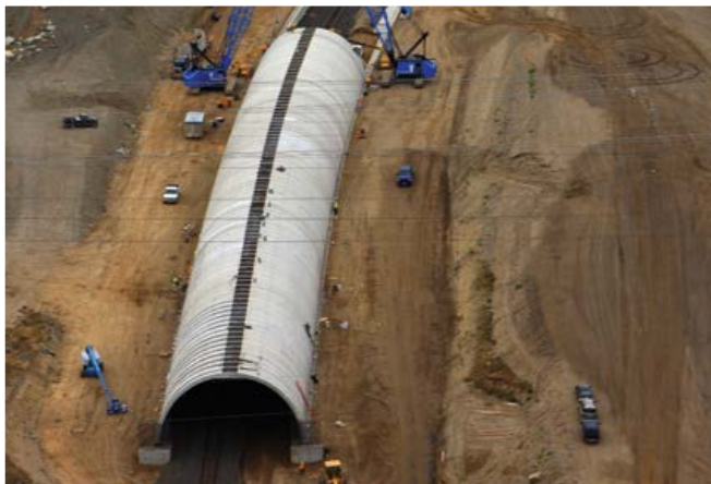
Ease of Installation – Precast modules allow railroad tracks to remain in service during construction.
