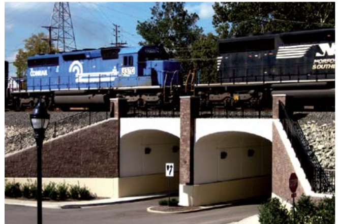
Railroad Overpass – Precast arch units support railroad loading over a roadway underpass.
