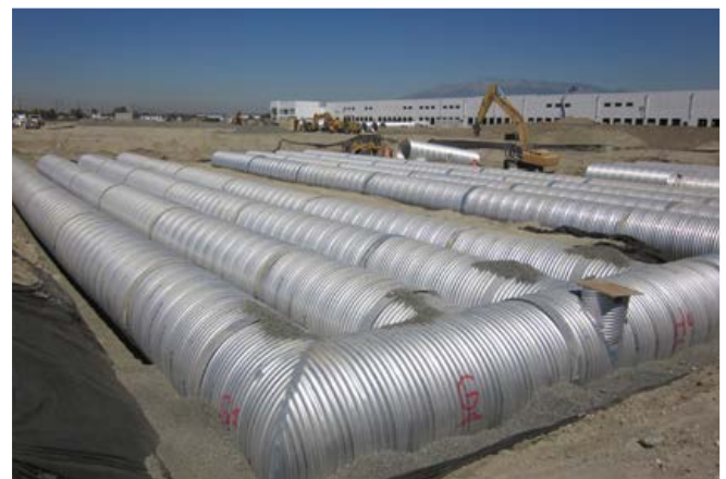
CMP Detention Systems are customizable and may be designed for heavy loading and high maximum cover.
