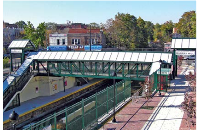
Skywalk Railway Overpass – Enclosed skywalk overpass carries pedestrian traffic over railroad.
