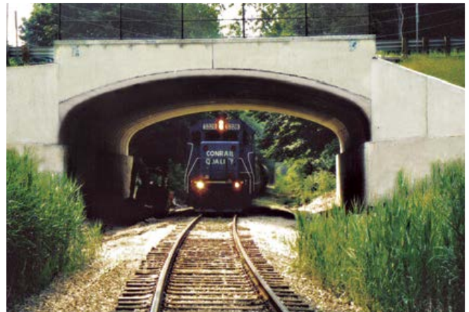
Railroad Underpass – Precast arch units provide a perfect solution to vehicular/pedestrian access roads over railways.
