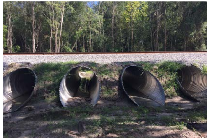
HEL-COR® ALT2 CMP was used to reline an existing timber beam bridge to avoid lengthy track down time and allow for a full structural repair.
