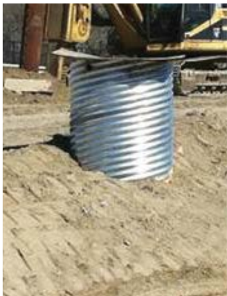
Liner Plate & CMP caissons for rail utility lines.
