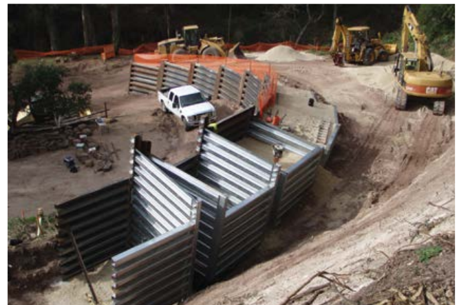
Retaining Walls – Bin-Wall is a lightweight steel that is easily assembled to fully enclose fill material for a solid wall solution.
