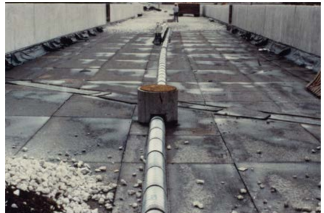
Use Contech Deck Drain to collect and transport water from the surface of the rail road bridge.
