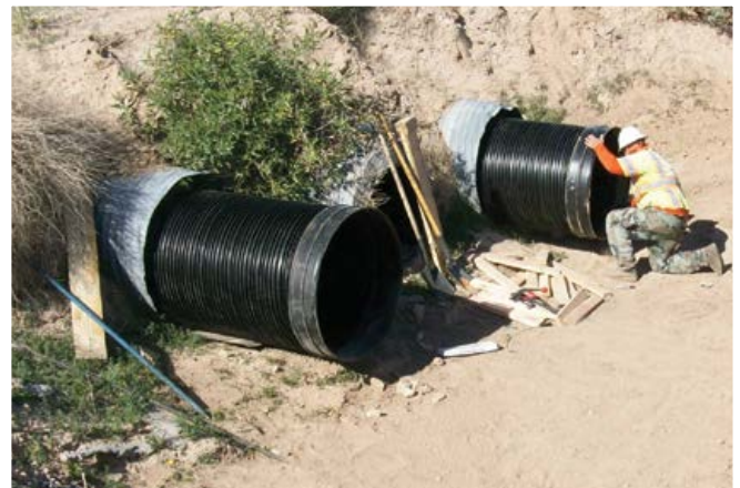
DuroMaxx® Steel Reinforced Polyethylene (SRPE) pipe is slip lined to provide a structural lining.
