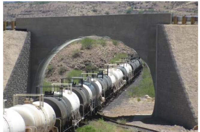
BridgeCor® structural plates unique corrugation allows for spans of up to 60 feet – ideal for railroad underpasses or large clearance areas.
