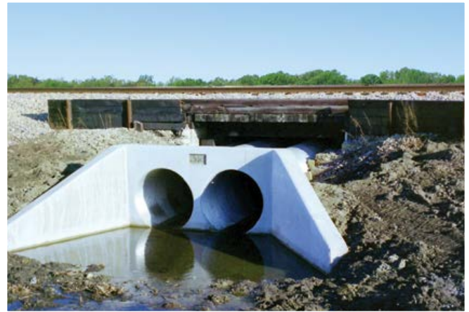
ULTRA FLO® corrugated metal pipe is often used to rehabilitate failing culverts and storm sewers.
