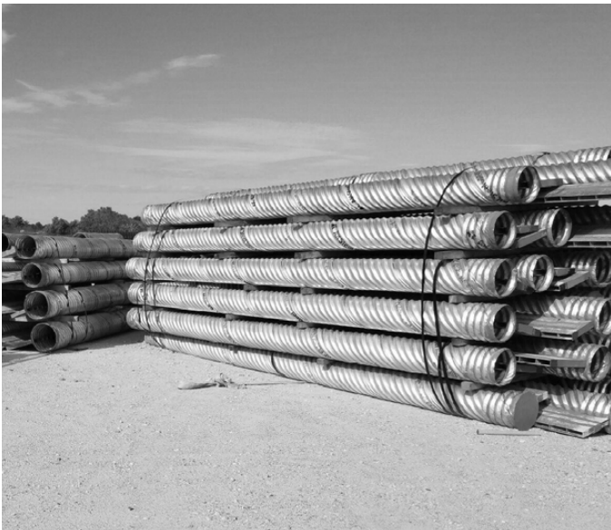
Slotted Drain shipped in bundles and stored on a project site.
