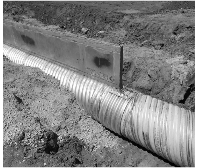
Connection of Slotted Drain™ System on to standard CMP.
