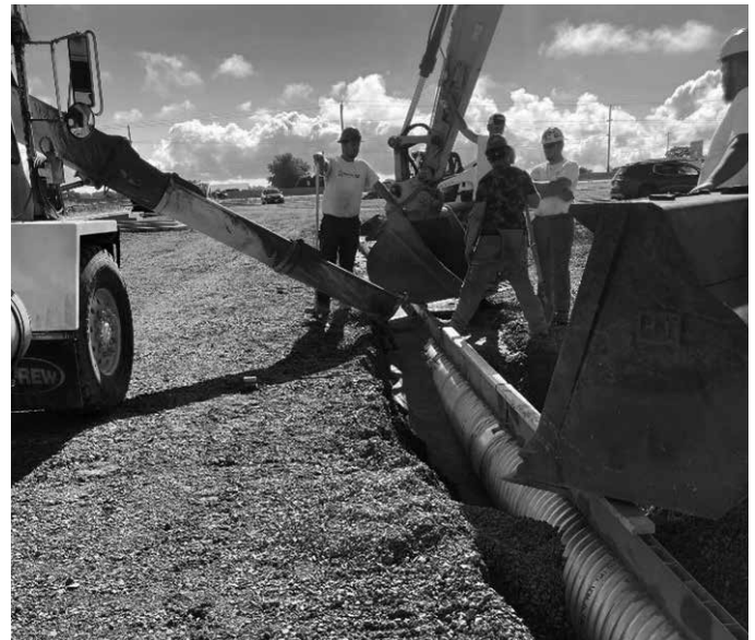
Flotation of the Slotted Drain™ System is a consideration during backfilling with a high slump concrete. A few of the many different techniques used to prevent flotation of the Slotted Drain include periodic placement of a low slump concrete on 10' centers before placement of the high slump concrete, backfilling in smaller lifts around the pipe, and restraining the pipe by various means.
