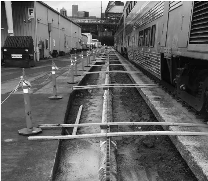
Flotation of the Slotted Drain™ System is a consideration during backfilling with a high slump concrete. A few of the many different techniques used to prevent flotation of the Slotted Drain include periodic placement of a low slump concrete on 10' centers before placement of the high slump concrete, backfilling in smaller lifts around the pipe, and restraining the pipe by various means.
