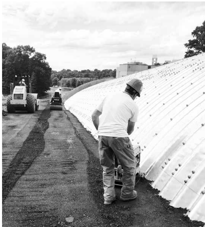
Figure 7. Adequate, uniform compaction is critical to building soil/steel structures.
