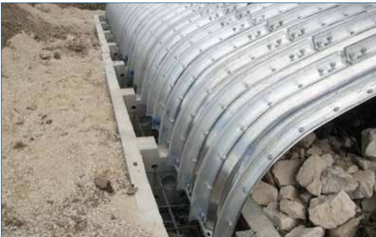
EXPRESS Foundations with Aluminum Box Culvert
