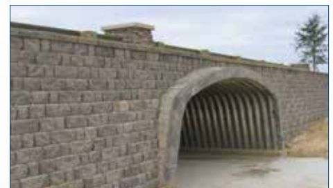
ALBC Pedestrian Underpass
