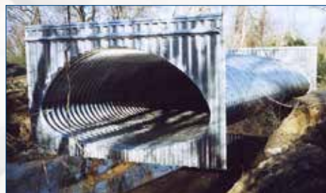
ALSP with Metal Headwalls
