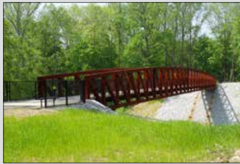
Vehicular & Pedestrian Truss Bridges
