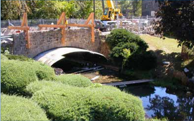
Reline with Aluminum Box Culvert
