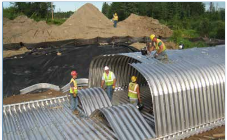
Easy Assembly with Aluminum Box Culvert
