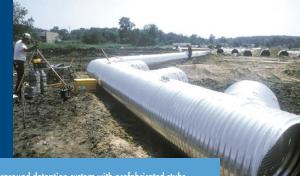
A CORLIX underground detention system with prefabricated stubs eliminates the need for forming concrete junction boxes.
