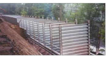
Application: Gravity-Type Retaining Walls for Rail
