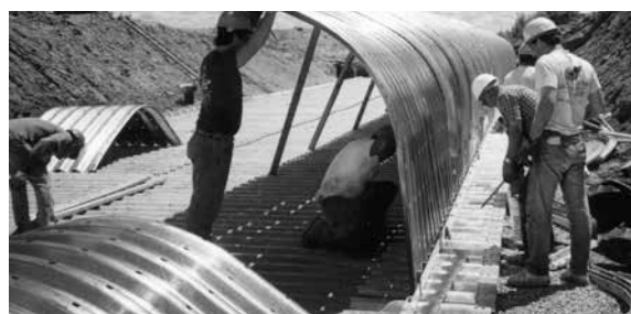
Assembly of ALBC Shell onto Full Invert
