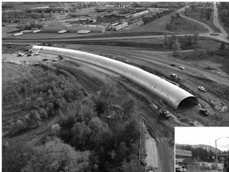
BridgeCor Tunnel Installation
