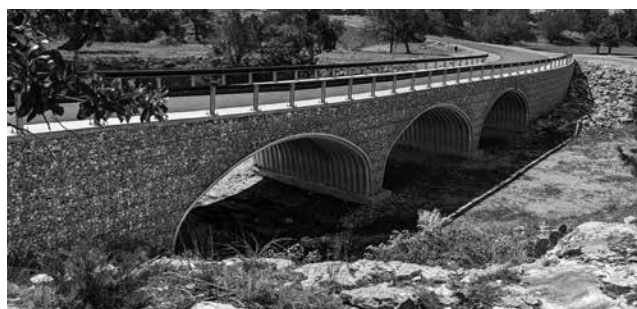
BridgeCor with Vist-A-Wall Welded Wire Wall System in Harper, TX.
