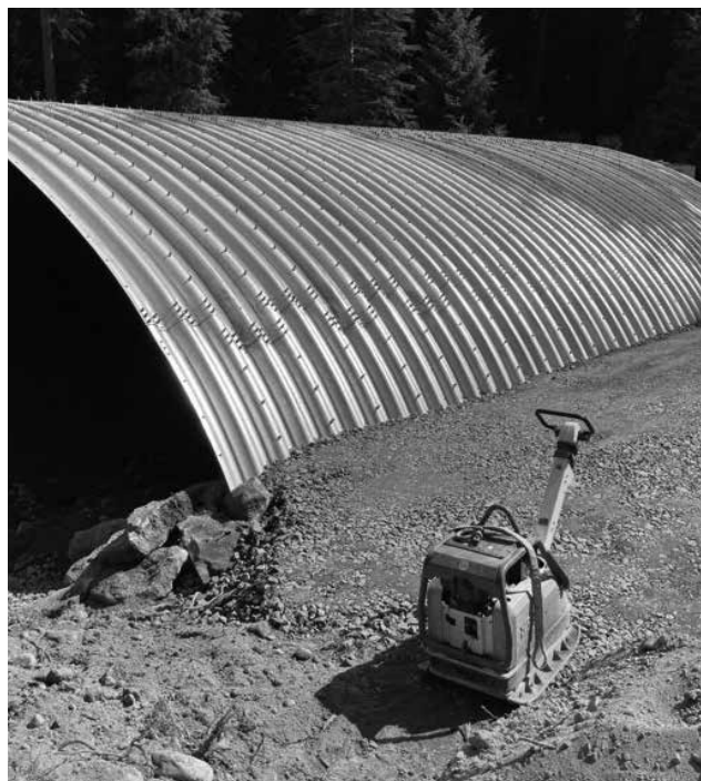
Each lift shall be compacted to a minimum 90% density per AASHTO T-180.
