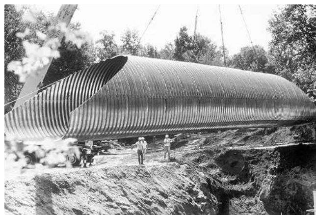
Lifting of Assembled Aluminum Pipe Arch
