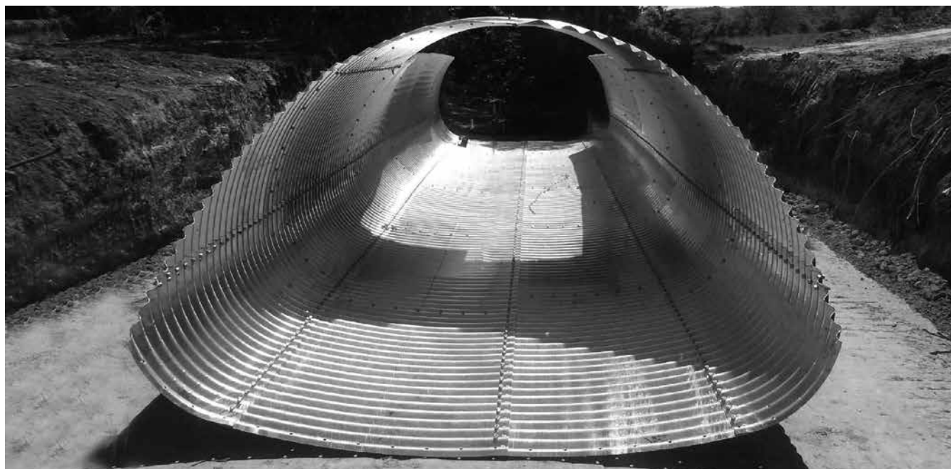
End view of an assembled MULTI-PLATE Pipe Arch
