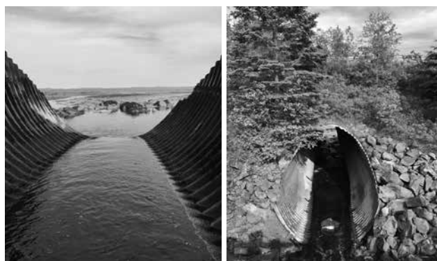
Bay of Fundy | Robinston, ME 52-Year-Old Aluminum Structural Plate Installed in 1966 | Inspected in 2018
