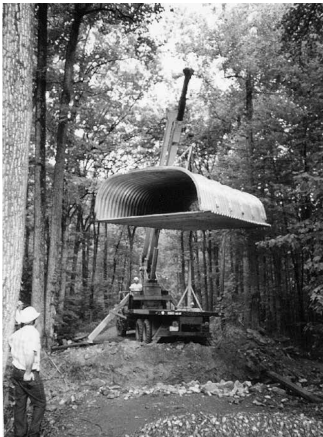
Lifting of Aluminum Box Culvert
