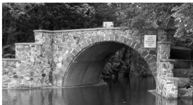
At the time of inspection in 2012, this Steel Structural Plate Single Radius Arch was 72-years-old. Installed c. 1940 | Inspected in 2012
