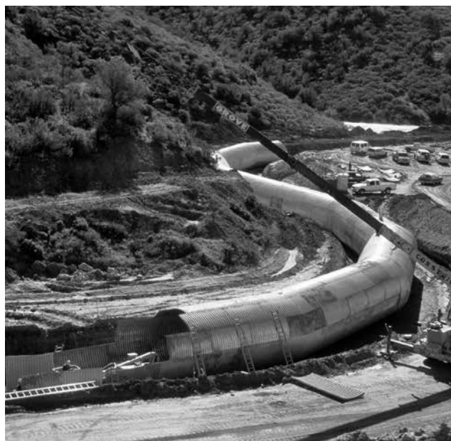
Along the Eastern Transportation Corridor in Orange County, California, this Key-Hole Slot MULTI-PLATE® structure was designed for the 115 ft. of cover.
