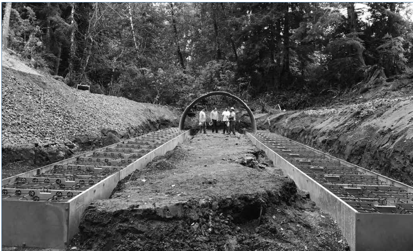
Steel EXPRESS Foundations are typically provided in unit length of 24'
