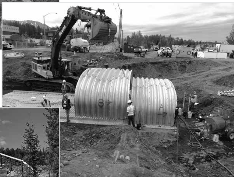
BridgeCor Box Culvert Assembly
