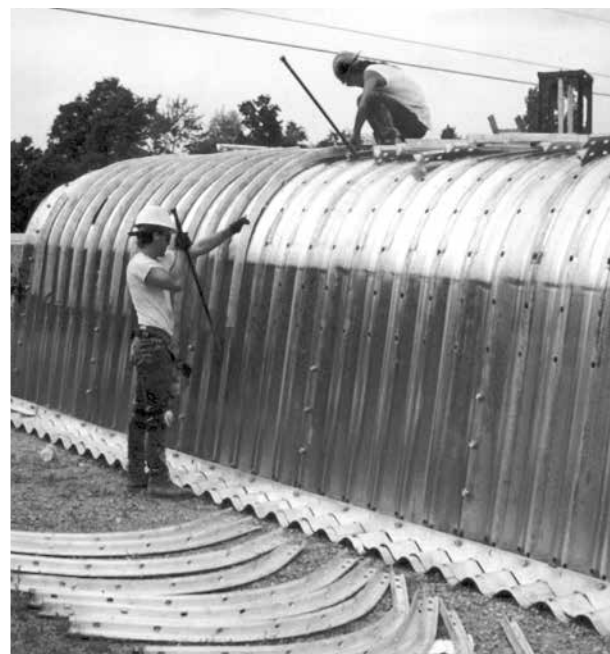
Installation of Ribs
