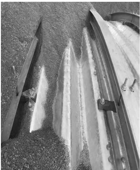
Typical External Rib System Assembly
