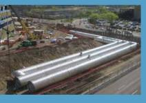
**U.S. Bank Stadium, Minneapolis, MN:** Being built downtown, there was limited footprint for stormwater storage. We worked with the engineer to design a 144" diameter perforated, corrugated metal pipe retention system that provided the required storage in a constrained footprint.
