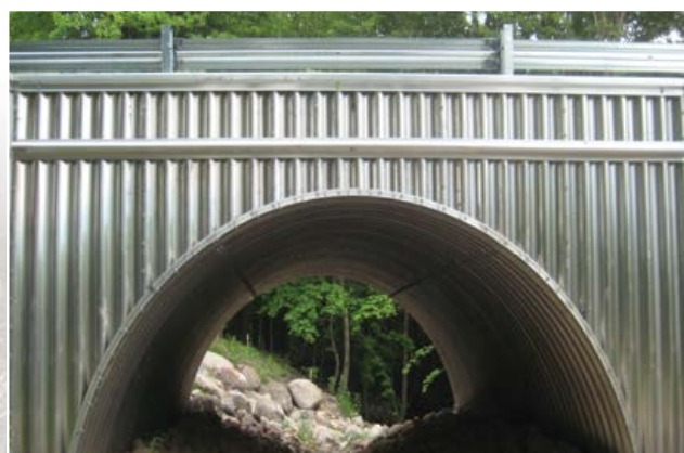
Aluminum Structural Plate with Headwall
