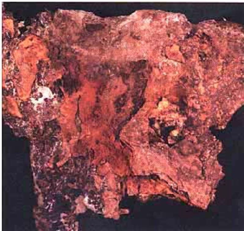
Galvanized Invert of end section
