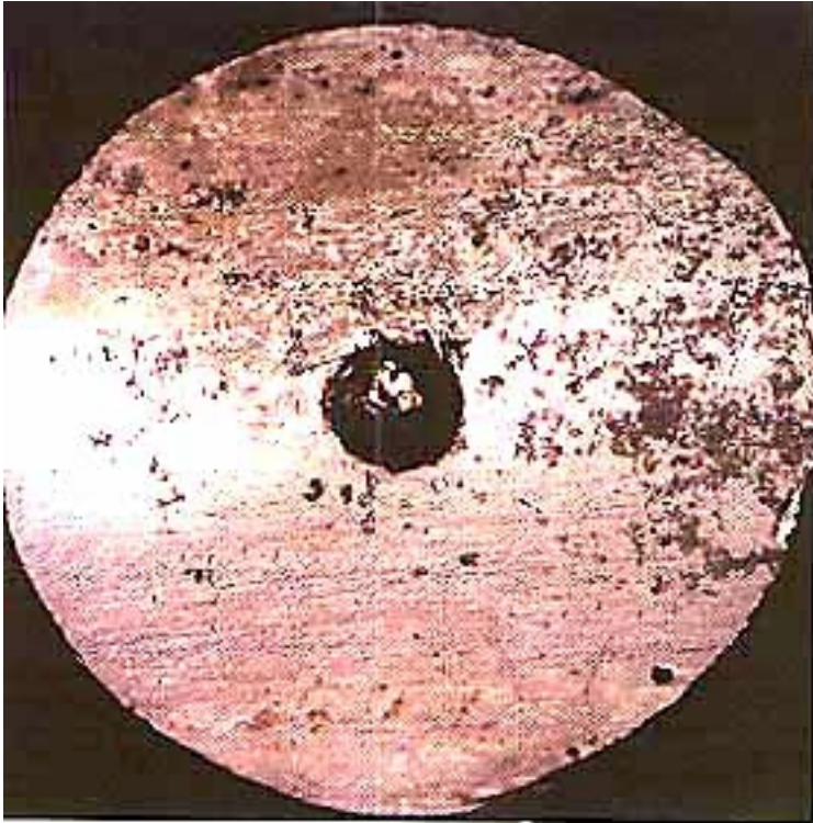
ALUMINIZED Type 2 Invert - Waterside
