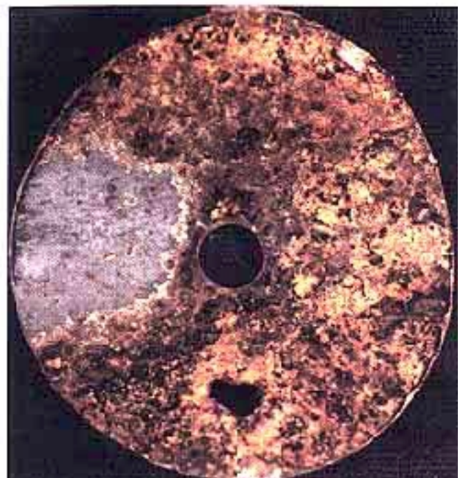
Galvanized Invert - Soilside
