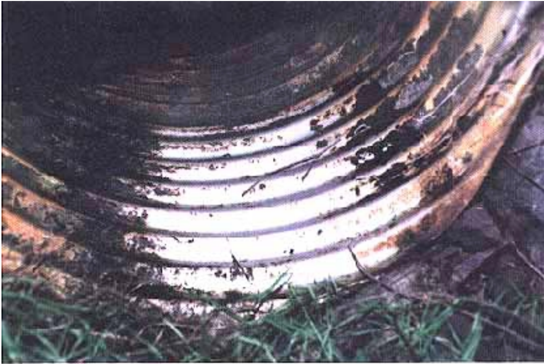
Snohomish County, WA 14-year-old ALUMINIZED Type 2 pipe is performing comparably with 42-year-old riveted Type 2 pipe with which it was joined in tandem 14 years ago.
