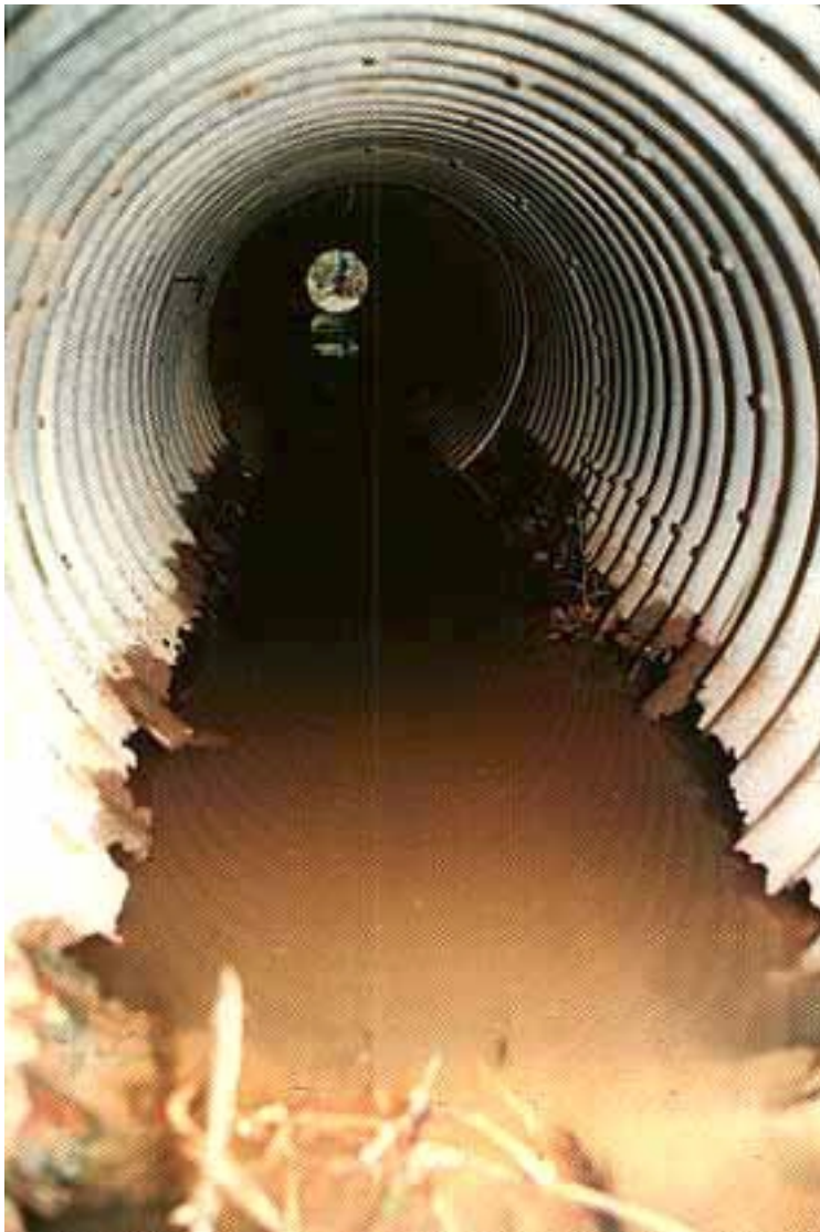
ALUMINIZED Type 2 - Invert - Waterside Mag. = 2X
