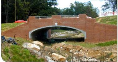
**Stream Restoration** – a three-sided structure replaces a deficient culvert causing stream pollution as part of a major renovation project to improve a main North Carolina waterway. The new clear span structure increases floodplain capacity and improves stream stability.
