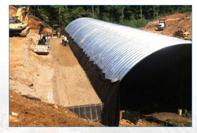
35'-8" x 17'-10" BridgeCor Backfill with Welded Wirewall – Gainesville, Georgia
