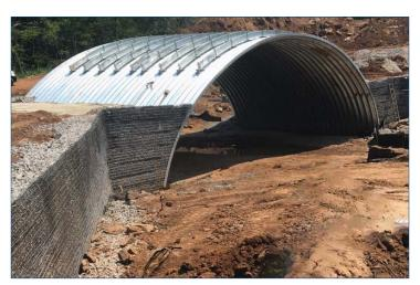
BridgeCor External Rib System (  $64^{\prime}\text{--}2^{\prime\prime}$  x  $19^{\prime}\text{--}7^{\prime\prime}$  ) during construction
