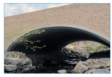
21'-2" x 10'-8" BridgeCor Arch with Keystone® Retaining Wall Systems - Shelton, Connecticut
