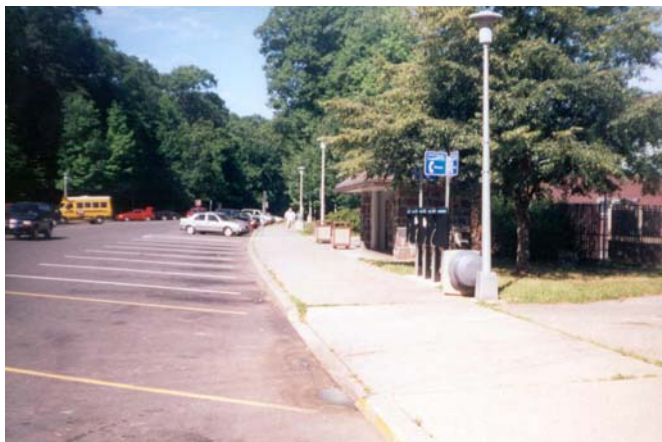
Figure 2 View of Lower Parking lot
