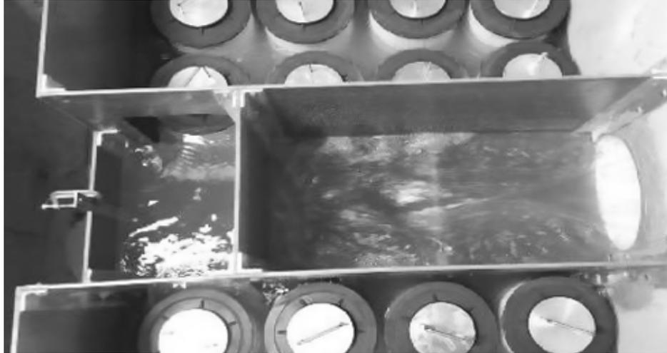
*3. Assess the condition of the filter cartridges and determine if cleaning is required.*
