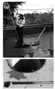
Inspection Utilizing Sediment Probe
